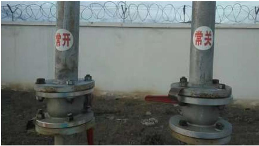
A photograph showing two industrial valves. The valve on the left has a red label with the Chinese characters '常开' (Normally Open). The valve on the right has a red label with the Chinese characters '常关' (Normally Closed). Both valves are mounted on a concrete base. In the background, there is a white wall topped with a single strand of barbed wire. |
